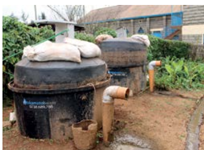
Biodigester Source: Takamoto Biogas
